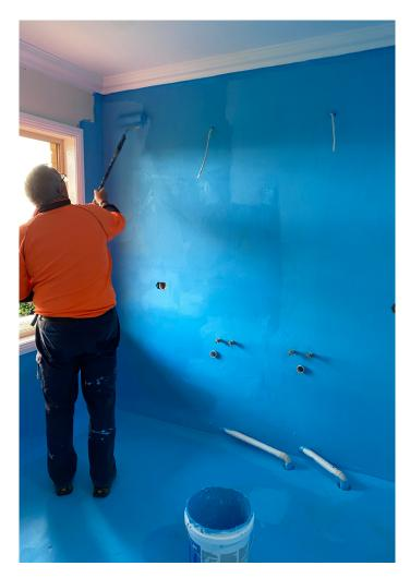
B&L Leakproof Deck and Shower, available from APTC Australia, is a Class III, low VOC, waterborne membrane system designed for use under tile finishes.
