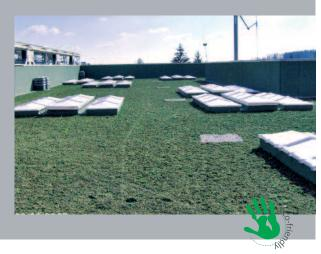
**PROJECT SPECIFICATIONS**: root-stop waterproofing finish in multi-layer systems for waterproofing garden roofs or decks with vegetation in contact with the structure to be protected.
